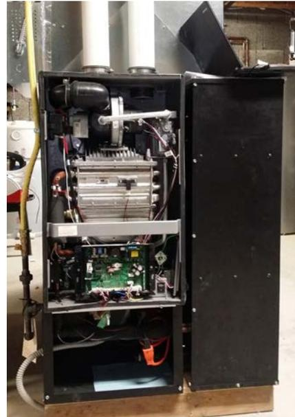
**IMAGE 1: iGEN i2 FURNACE WITH COVER REMOVED**
